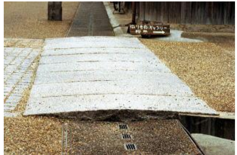
Stone bridge over the ditch
