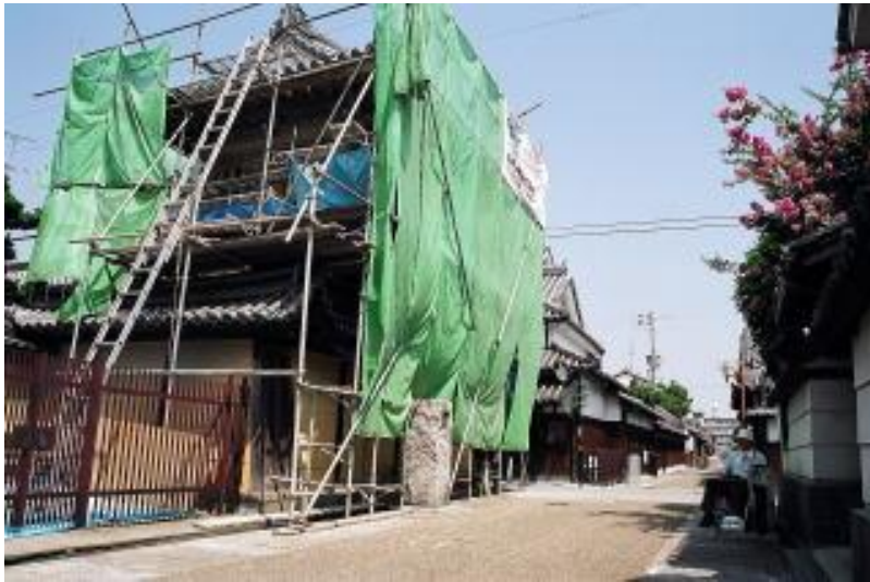
Bell Tower (Under Repair)
