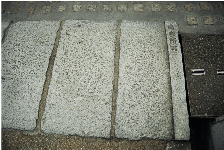
Ditch water for fire fighting
